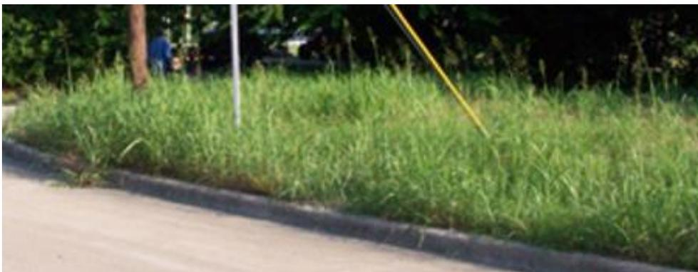
High grass can also obscure the shoulder. Shoulder and roadside maintenance such as grading or mowing should be done to define the edge of shoulder and ditch so that motorists can see the shape, condition, and limits of the roadside.
